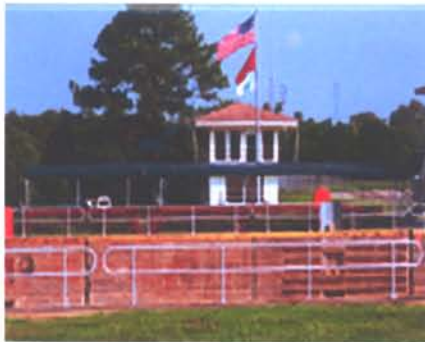
Algiers Locks/Intracoastal Canal
